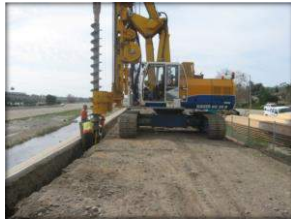
Repair at San Juan Creek, Orange County
