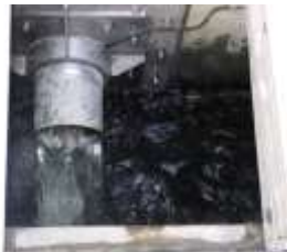
Appearance of the effluent
