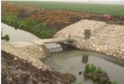
Final screening and drain bank protection work
